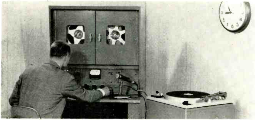
Recording unit handles microphone, phono and self-contained control-tone generators
